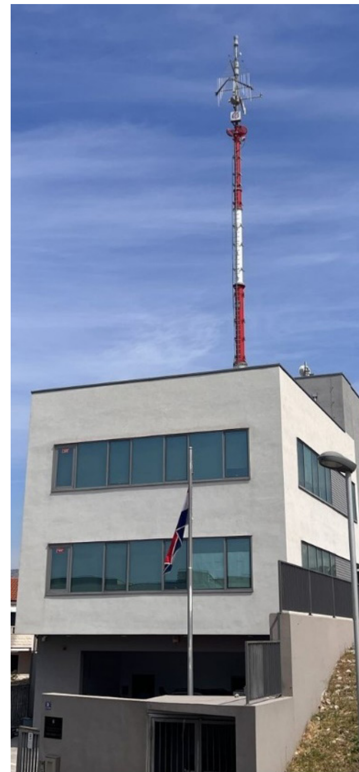
Figure 5.5 New antenna pole at the control and measuring centre Split
