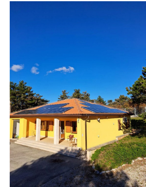
Slika 5.7 New solar energy station at the control and measuring centre Rijeka
